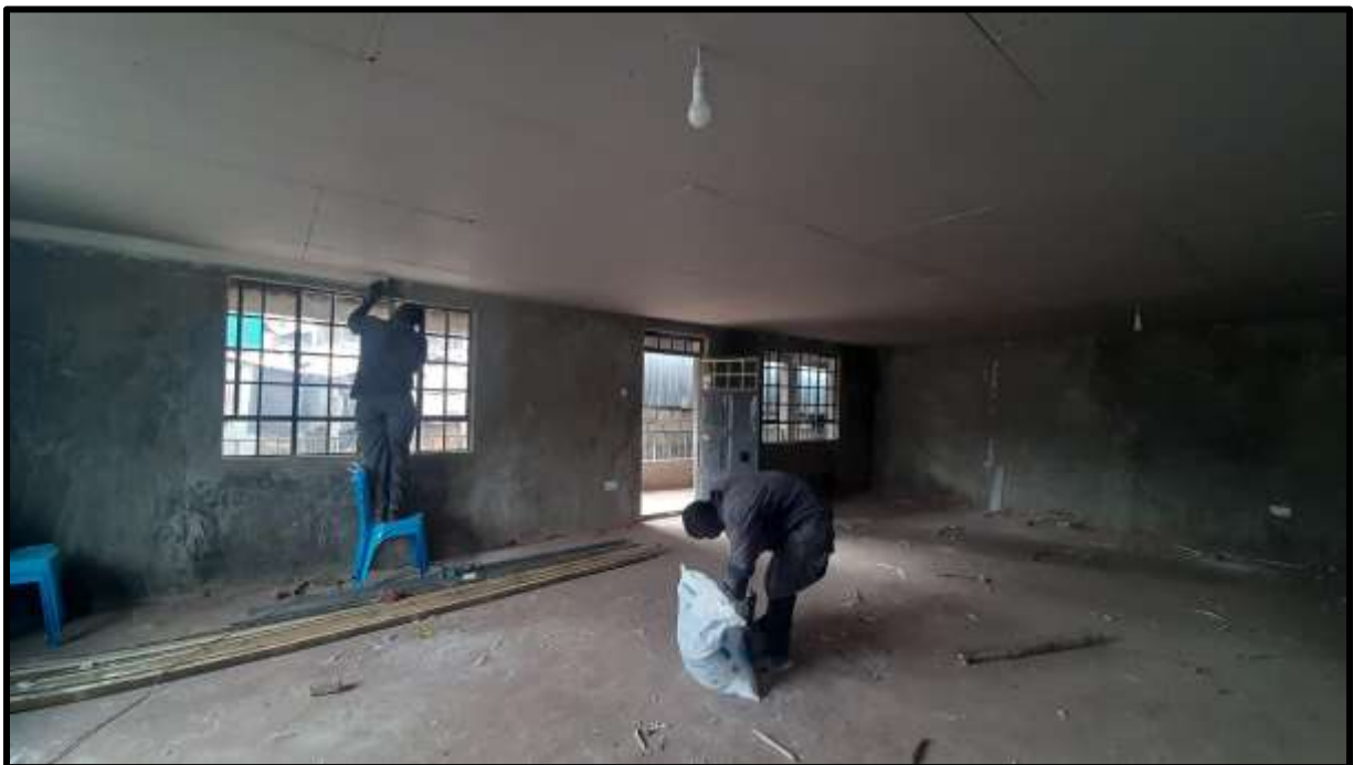
Ceilings and lights connected (End of May 2021)
