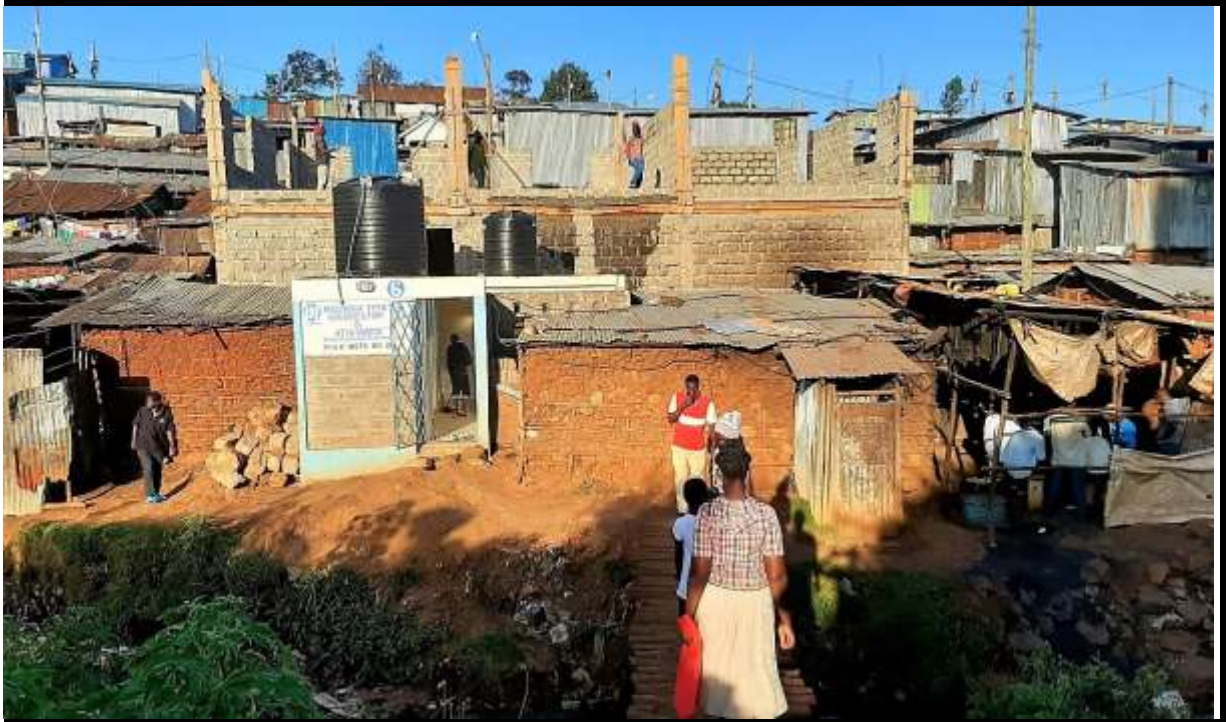
The first floor is almost accomplished (early December 2020)
