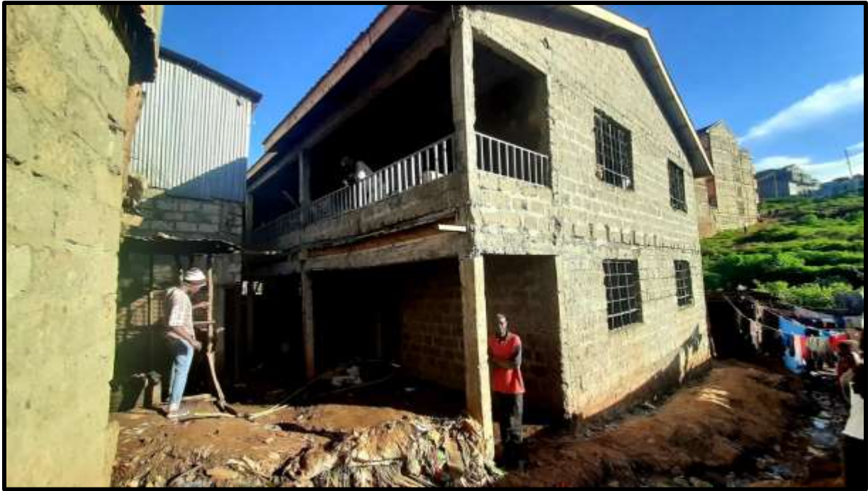
A terrace is made on top floor (Mid April 2021)
