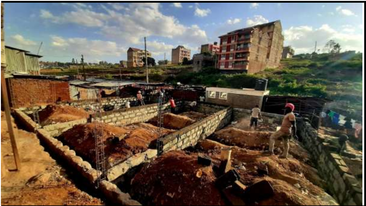
Foundations are put in place (End of September 2020)
