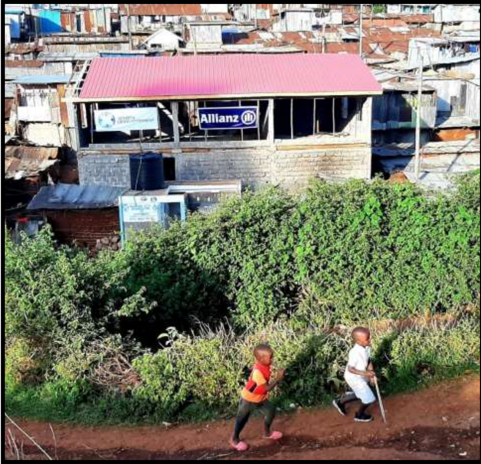
The tiled roof is fixed (early February 2021)
