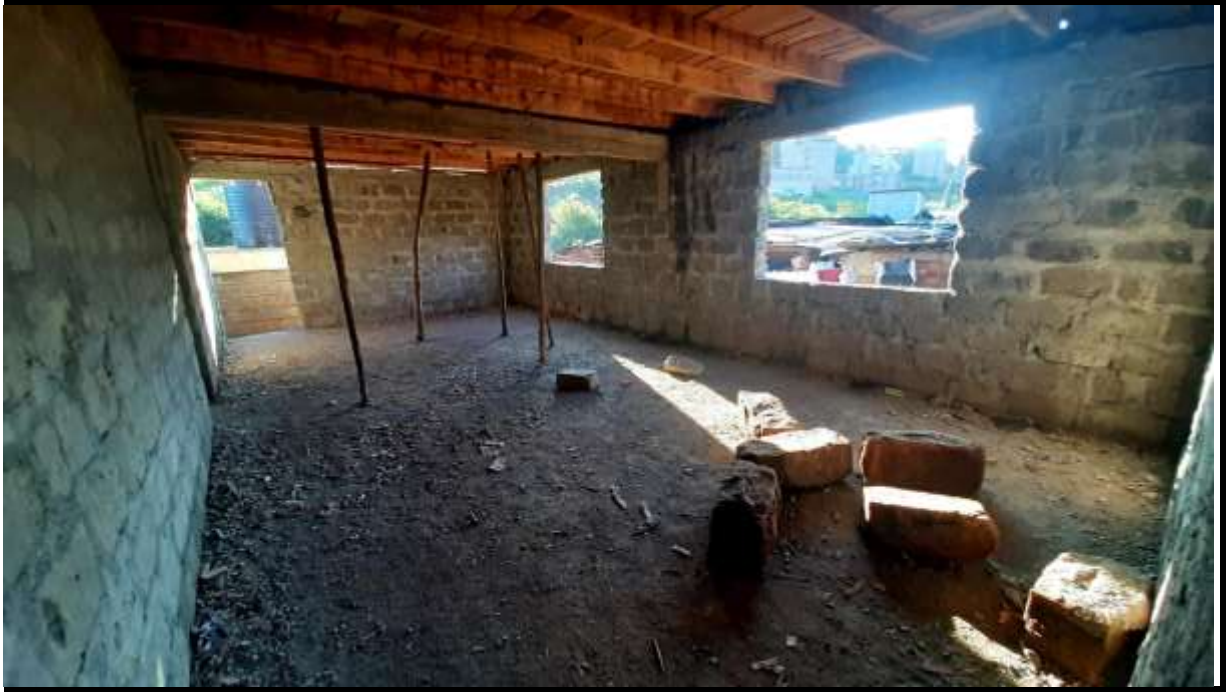
Inside one classroom (Mid November 2020)
