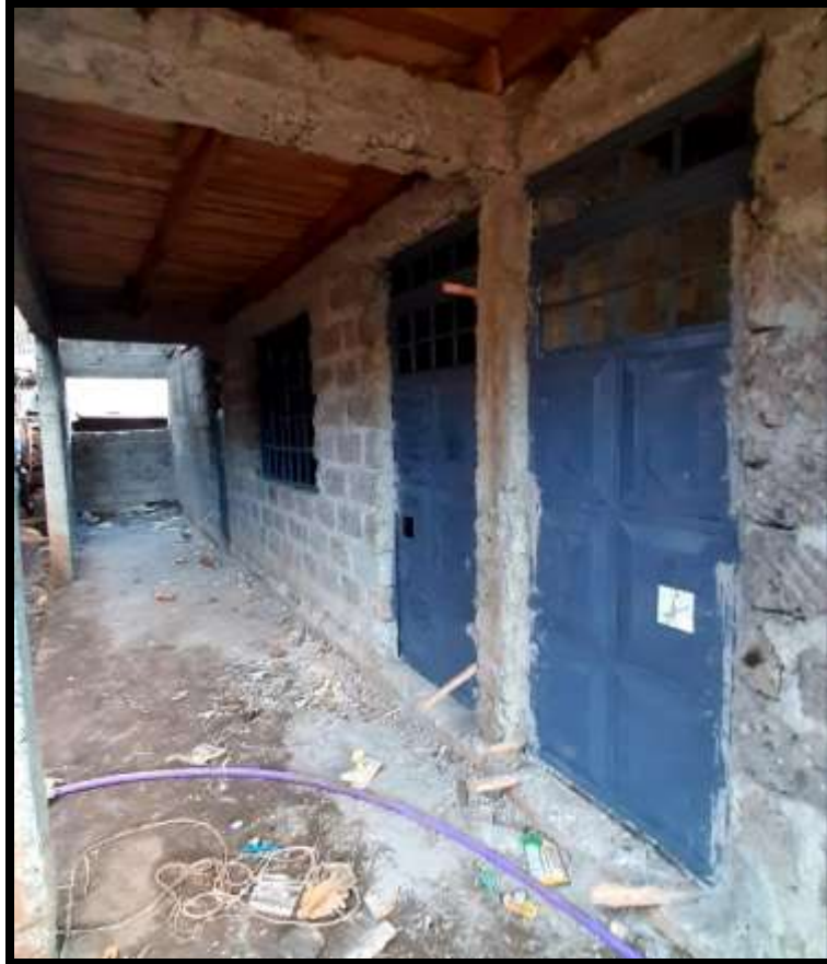
Doors and windows fixed (end of February 2021)
