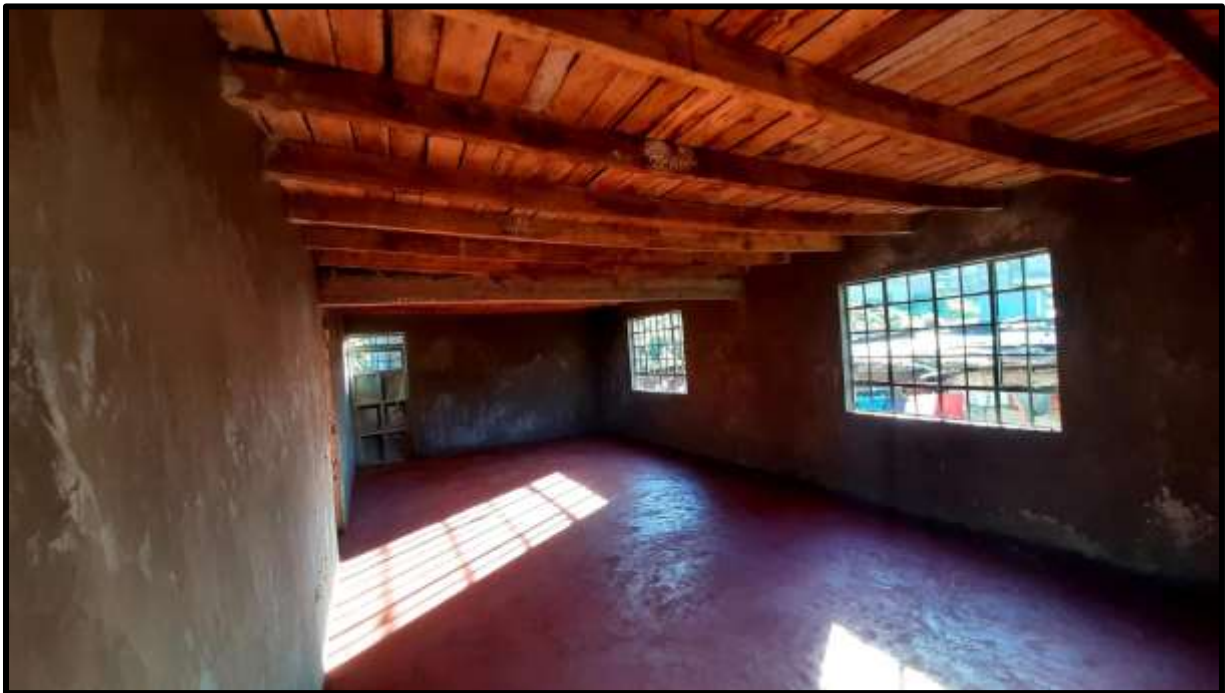
Plastering of walls inside the rooms (End of April 2021)
