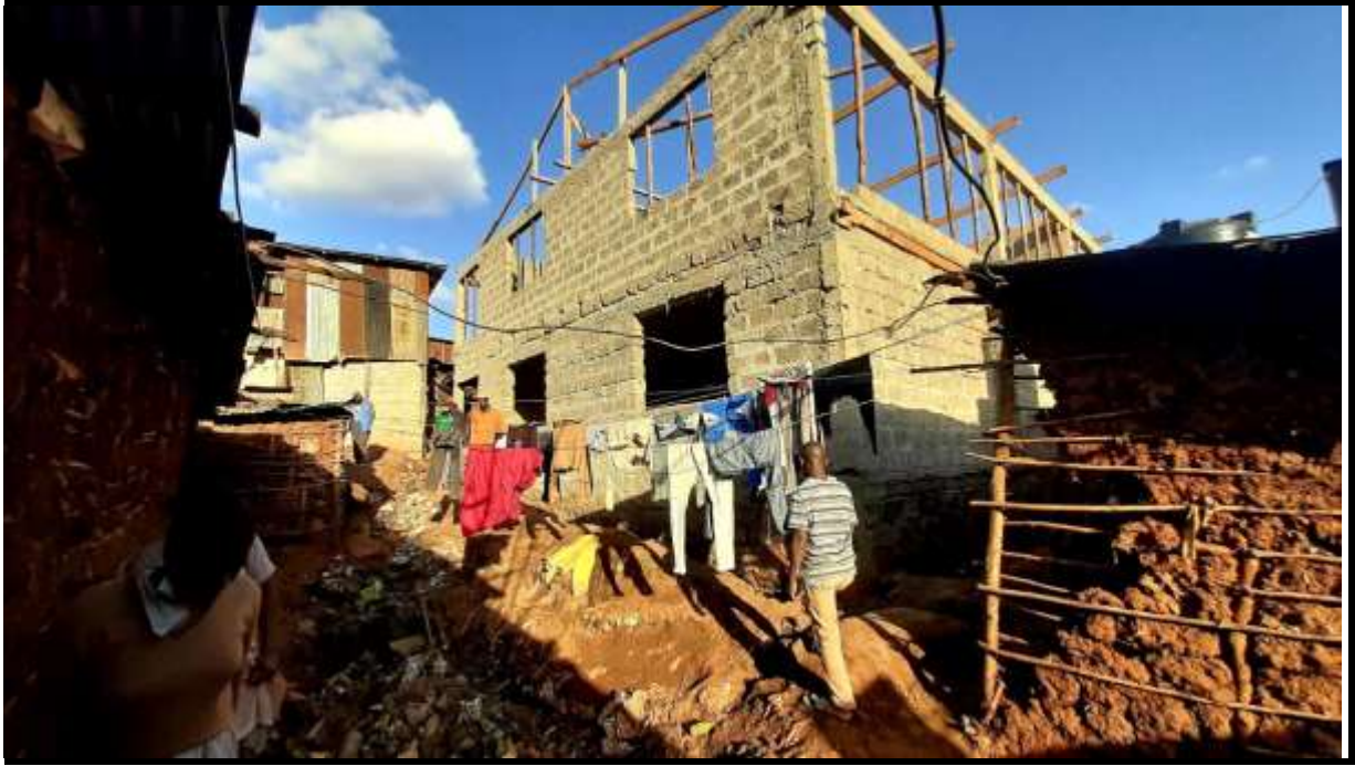
Top floor and roofing in progress (Mid December 2020)
