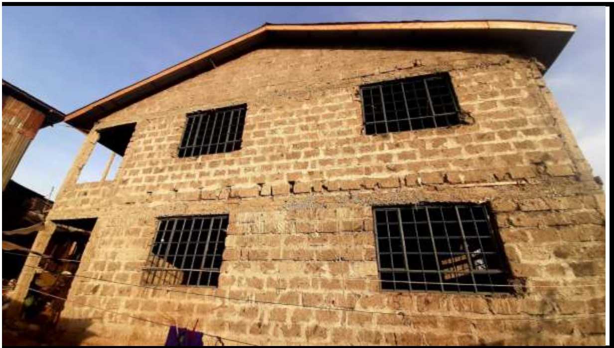
One of the side wall (end of February 2021)
