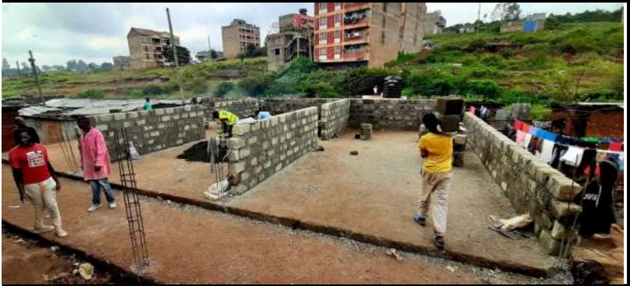
The walls of the groundfloor are raising up (Mid October 2020)
