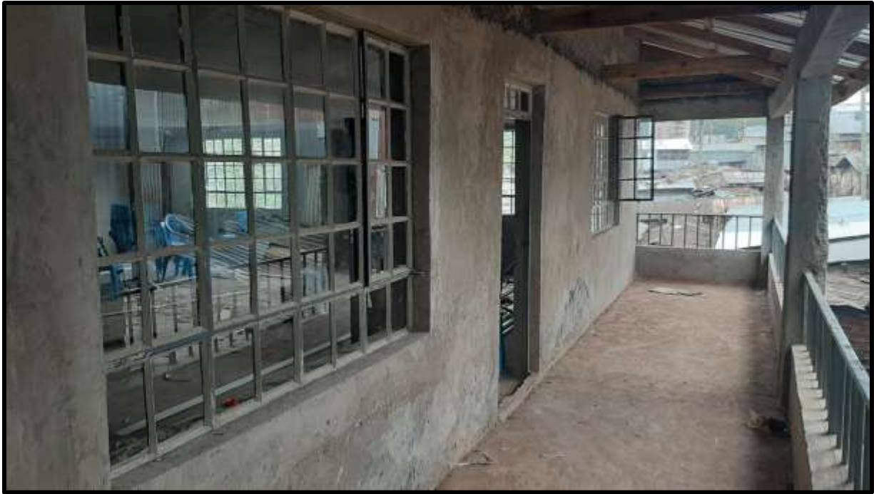
Glass windows and inner doors fixed (Mid May 2021)
